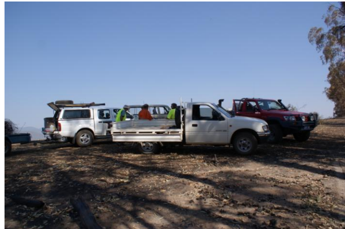
Taking a break whilst removing the old fence line.
